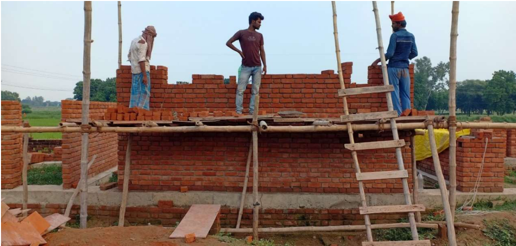
Working on the east interior wall
